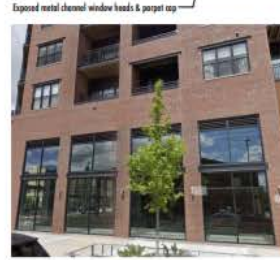
Exposed metal channel window heads & parapet cap
